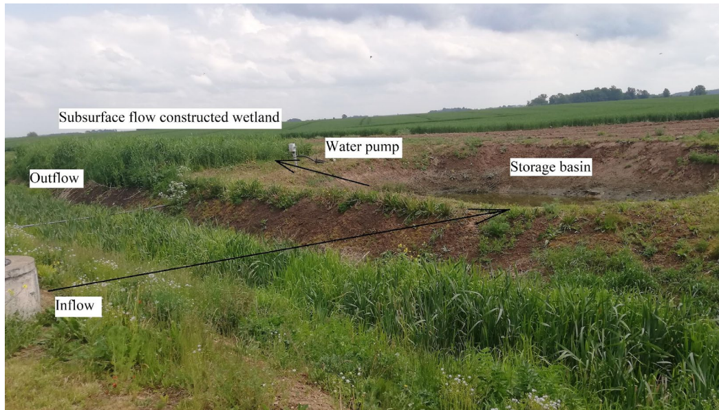
Fig. 2. A storm water treatment system with horizontal subsurface slow constructed wetland at the Mezaciruli farm. Photograph taken by the author.
